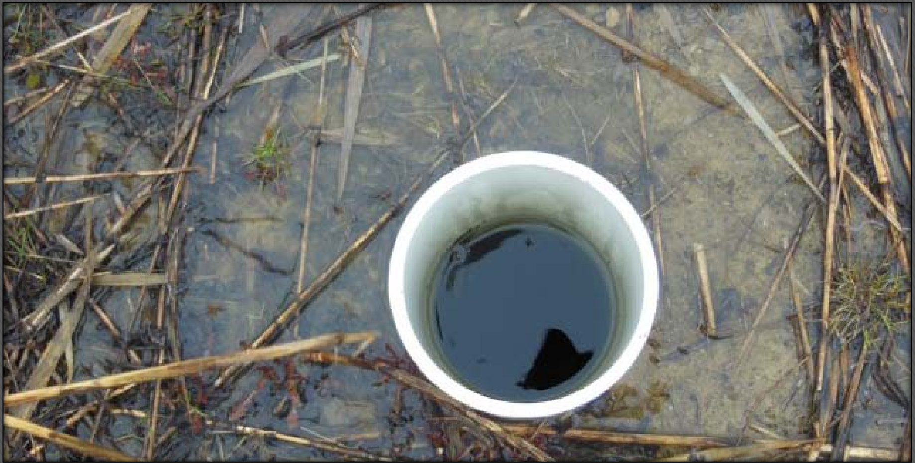
Uncapped water well on site. Shultz Well, Sanilac County
