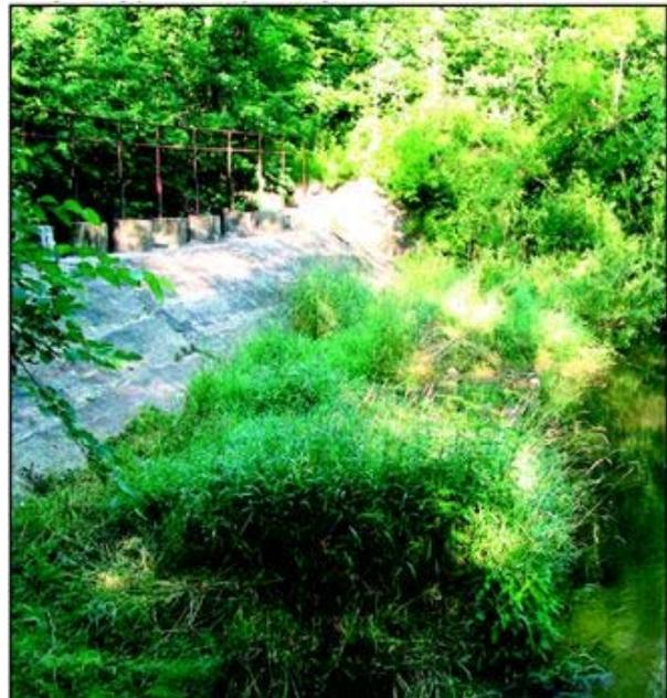
**DAM TO BE GONE** – The “upper” dam on the Paw Paw River built at the turn of the 20<sup>th</sup> century to divert water to the Watervliet Paper Mill will be removed, restoring the original course of the river through Hays Park. The dam leaks water underneath and around it, allowing a trickle of water to flow in the old riverbed. At flood stage on the river, water flows over the top of the dam.
