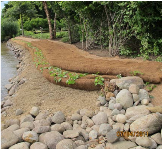
BioD-Block soil lift system for shoreline protection
