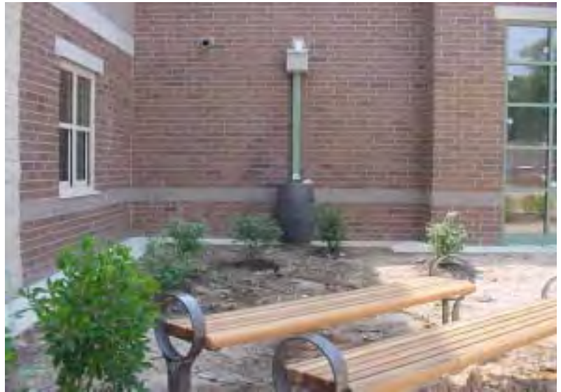
Rain barrel in use at a school (Photo: Low Impact Development Center)
