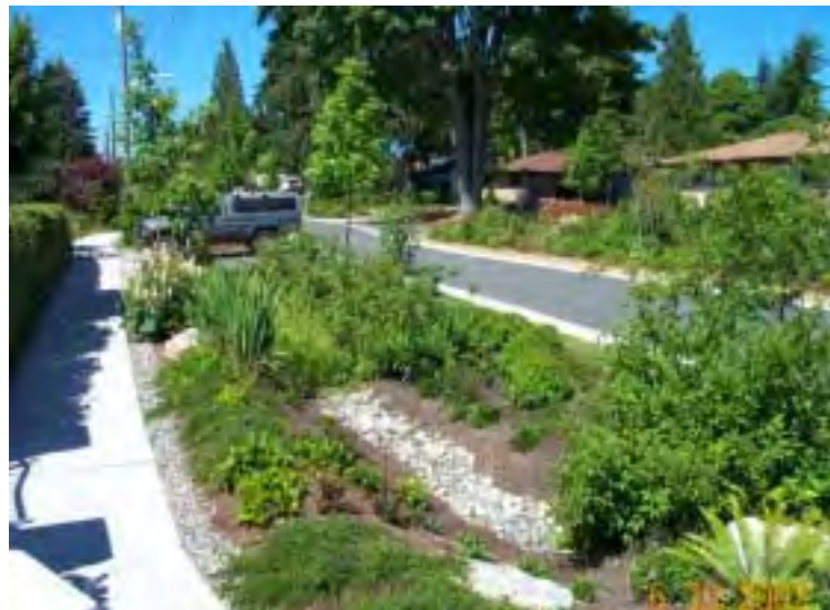
Street-side swales can dramatically reduce stormwater runoff from roads (Photo: Seattle Public Utilities)
