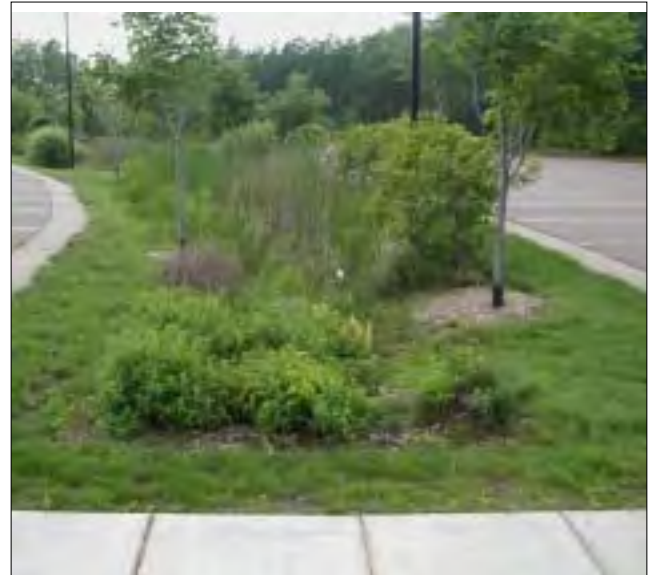
A vegetated dry swale (Photo: Applied Ecological Services)
