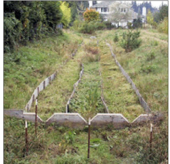
Wet swale with weirs to conduct flow research (Photo: Center for Water and Watershed Studies)
