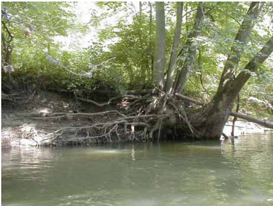
Figure 22: Undercutting of tree roots along the South Branch
