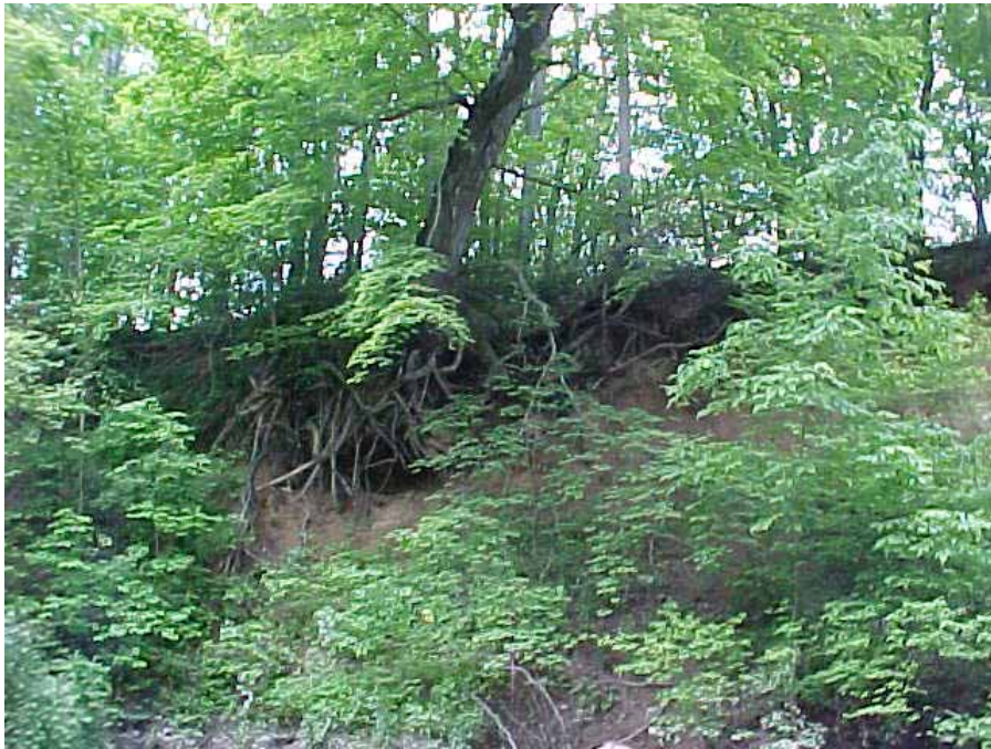
Figure 21: High, eroding bank along the South Branch
