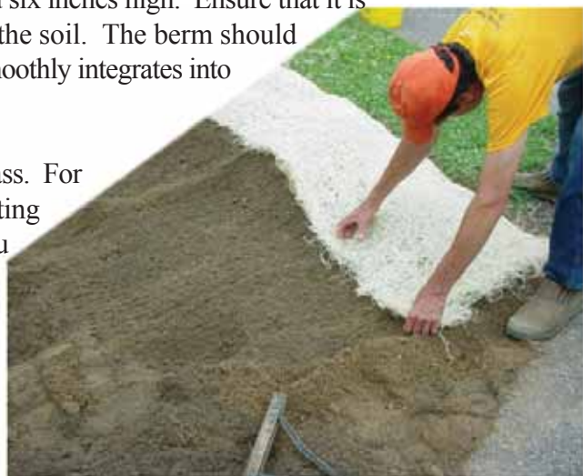
Erosion control matting made of coconut fiber is carefully placed along the berm to prevent erosion on the down hill side of the rain garden.
